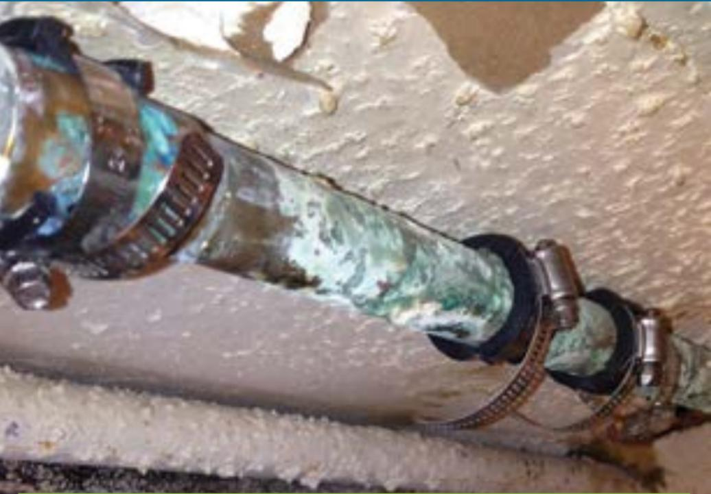
A clamped pipe is a temporary solution to stopping pinhole leaks. Anti-corrosives, including sodium silicates, help provide lasting protection from pinhole leaks.
